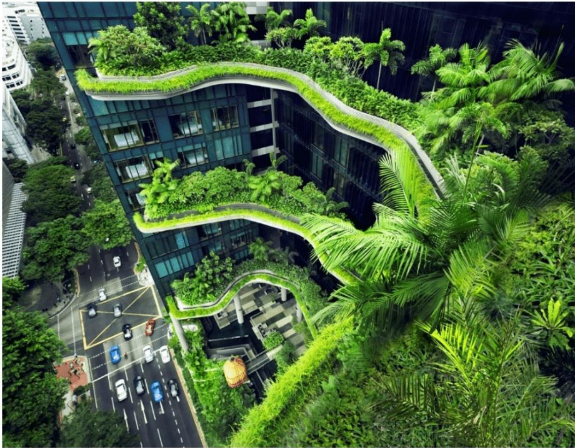
Figure 1 - Urban green spaces in Singapore - Aerial view
